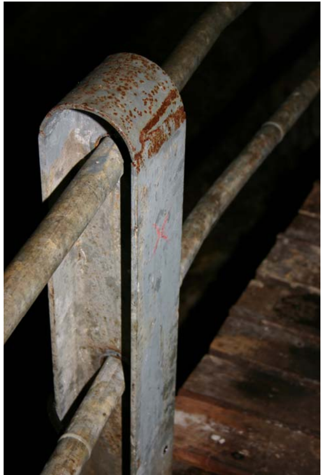
Infrastructure in Clearwater Cave.
